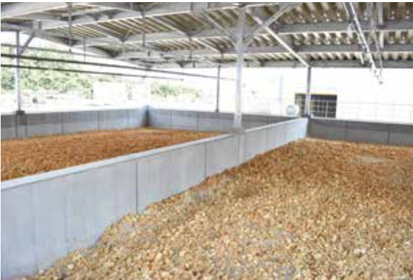
Deodorization equipment at the Iga Recycle Center composting facility
