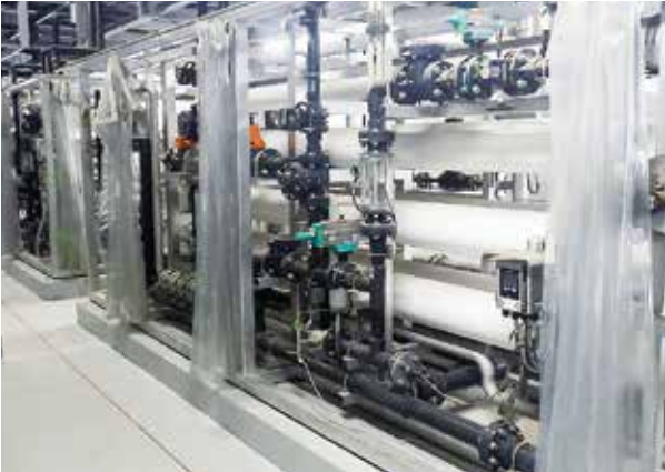
RO membrane treatment equipment at water treatment facility at Mie Recycle Center
