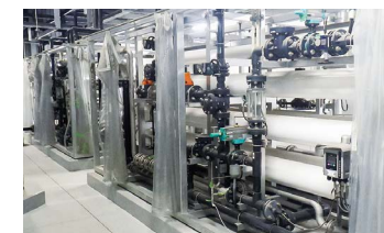
Mie Recycle Center to recycle water resources Reverse osmosis (RO) membrane treatment equipment in the water treatment facility
